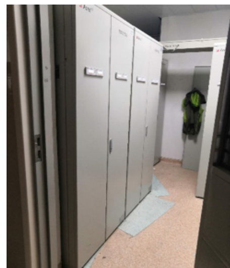
(2) Site Installation Picture
